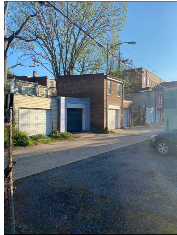
03 VIEW, EAST FROM ALLEY
